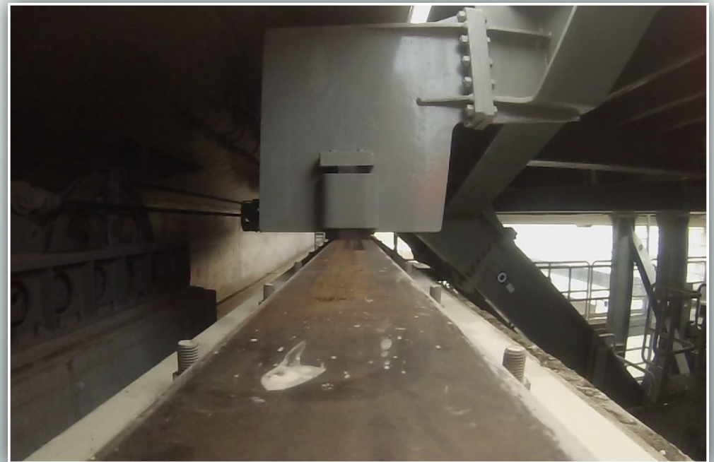
Lunac 2+ applied to the new Panama main lock door rail system after 3 years, to prevent the system from corrosion and especially adhesive wear (25 mm side shift during filling locks and earthquakes). Vertical load during lateral movement: up to 975 kN. Wheel-pressure up to 560 MPa.
