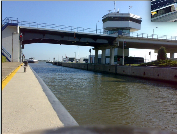
Houtribsluizen (Lelystad) L2+D coated lock gate hinges.
